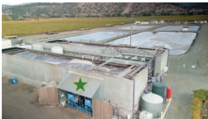
FIGURE 1 Sutter Home Winery ran trials at its wastewater treatment facility. The green star shows Recovered Water Solutions' trial space.
